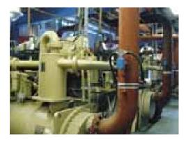
A bank of vapour compressor chillers bring the current chilling output to 8MW. Photo:  $\ensuremath{\mathsf{MG}}$
